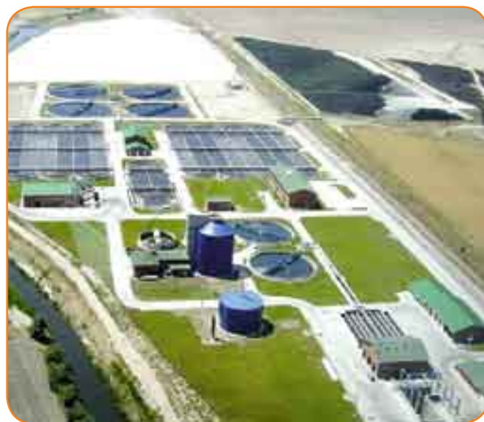
This sewage treatment plant ensures better health in Diyarbakir.
