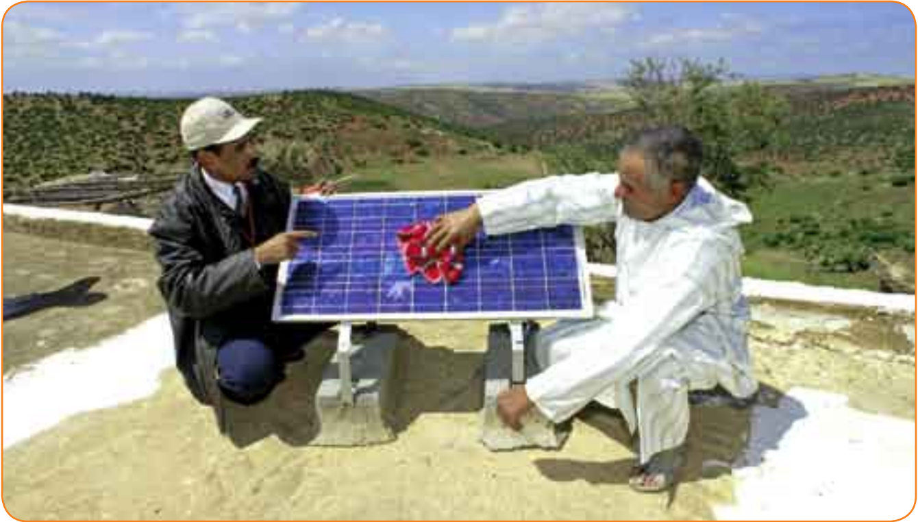
Promoting regenerative energies – photovoltaics in Morocco.
