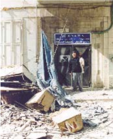
Nablus office after "operation defensive shield"
